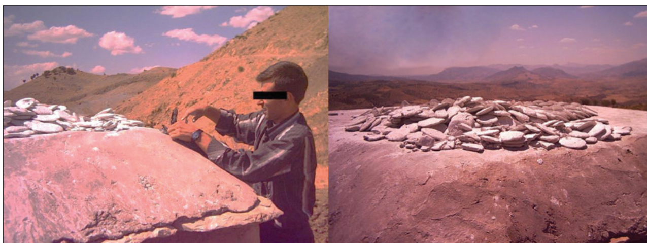
Figure 8. The white soil is laid on the roofs for drying. It will be used when necessary. Pay attention to the roof cover. A typical example of white soil cover (The archive of Dr. A. Şenyiğit)
