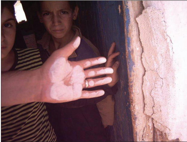
Figure 11. White soil plastered on the wall easily adheres to the existing material (The archive of Dr. A. Şenyiğit)
