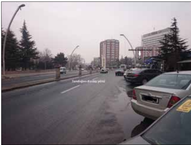
Figure 4. Picture of Tandoğan Intersection Döğol Street
